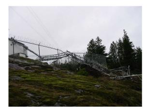
VE7BEU, the wind folded the 88 foot tower, requiring it to be cut down at the base to protect other towers at the site. Since replacing the original 88 foot tower will require up to a year, the current plan is to use some temporary antennas on makeshift poles or mounts to get back on the air. A new tower will be rush ordered and installed on the existing base. The new tower would be self-supporting and very strong at 48 feet with minimal antennas.
